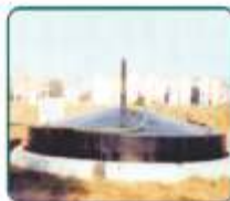
Renewable Energy Biogas Plant
